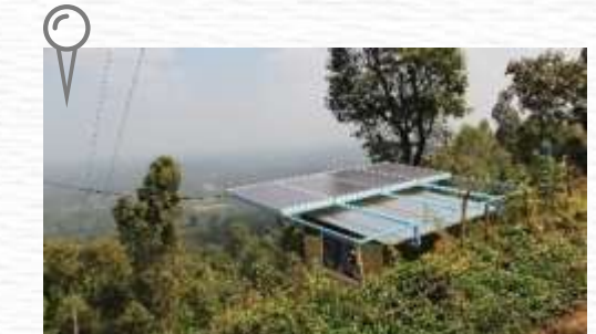
Amrita Sphuranam : Rural Electrification using solar Power
